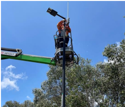
Image: Central Management System gateway install, Caloundra
