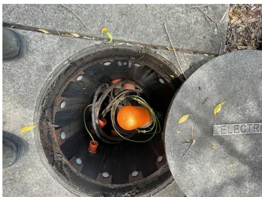
Image: Circular Electrical pit with cable junction
