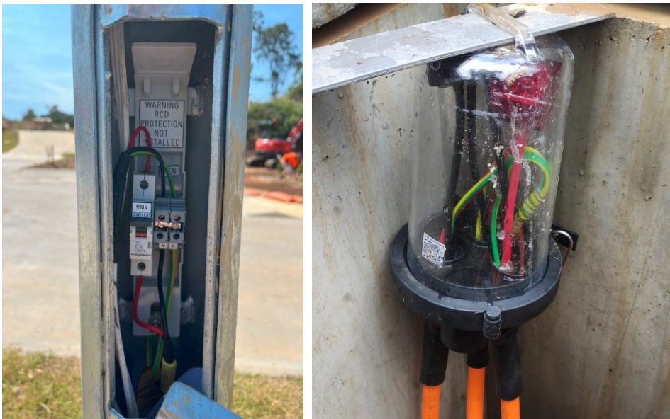
Image: In pole equipment and underground joint
