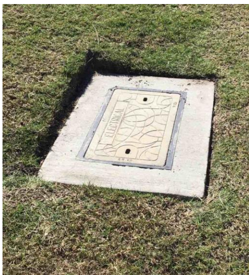
Image: Electrical pit with concrete collar
