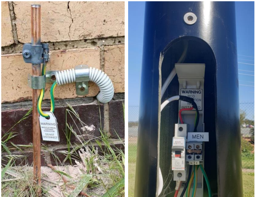
Image: Earth stake and in-pole M.E.N
